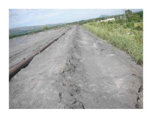
**Result:** The entire tailings complex was treated creating a light crust over the surface, which will prevent the formation of erosion channels caused from heavy rains, allowed for the integrity of the tailings to remain untouched, eliminated the use of an expensive and inefficient sprinkler system and most importantly prevents dust meeting all environmental requirements, improving community relations and providing a safer and healthier work environment.
